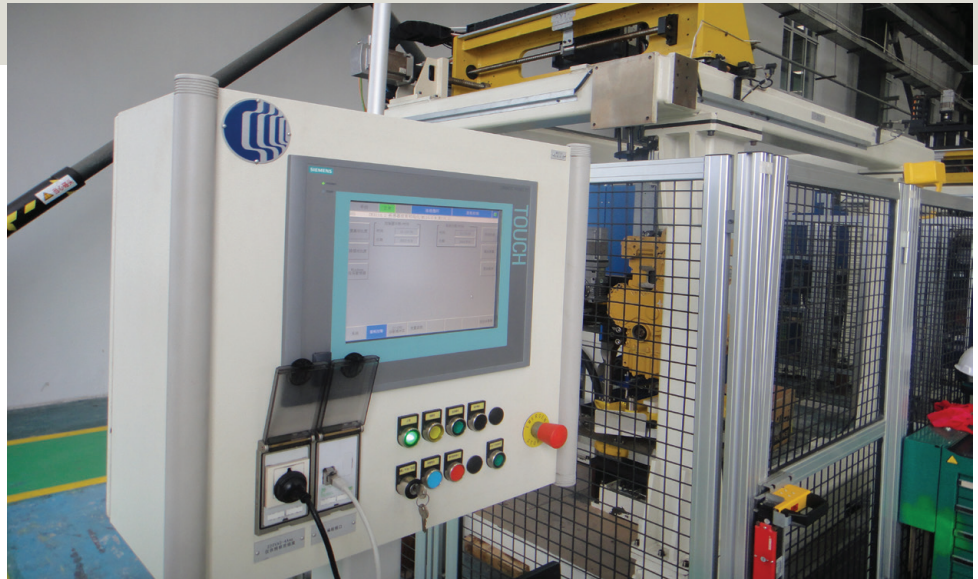
Process Simulate Virtual Commissioning is used to troubleshoot cell controller program.
